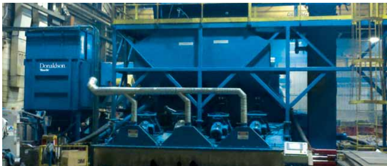
VH 2-12 on Blasting
